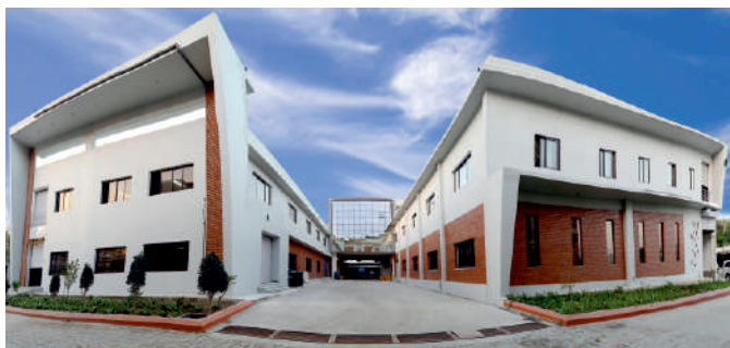
Tempsens Instruments U# II Cable Plant
