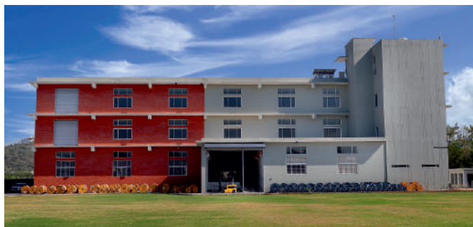
Tempsens Instruments U# IV Cable Plant
